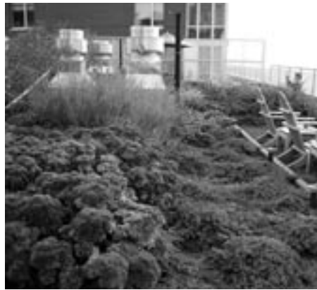
How does your garden grow? An intensive green roof atop the environmentally friendly Solaire building in Battery Park City.
